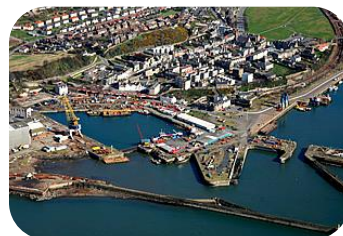
New Build Fabrication
